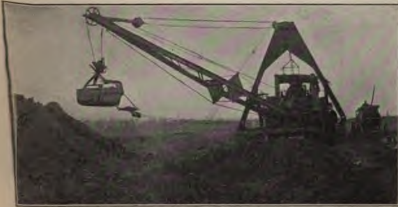
Avery Traction Shovel Excavating a Drainage Ditch.
